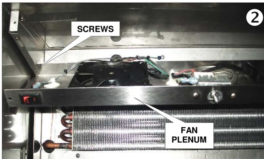
Tilt the fan plenum forward and remove the RANCO Thermostat mounting screws.
